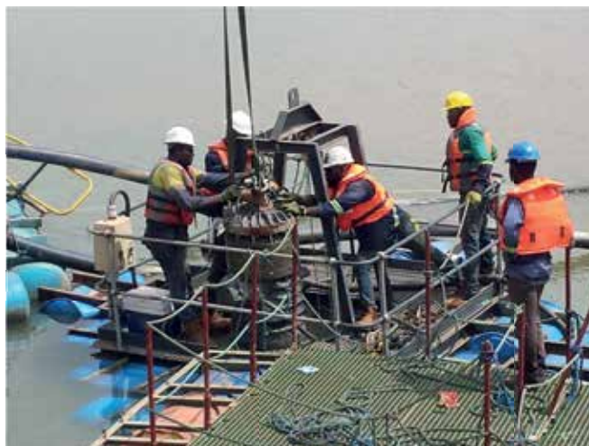
Jenny J90H being installed in a tailings dam
